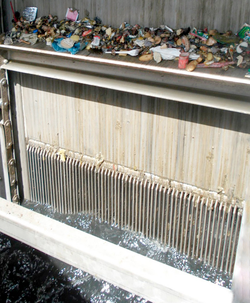
HUBER Coarse Screen for protection of pumps for sewage water lifting.
