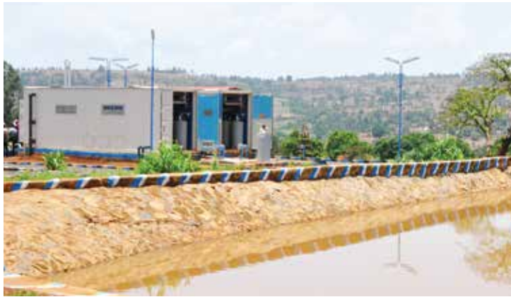
Bako Potable Water Treatment Plant 40,000 People, Ethiopia
