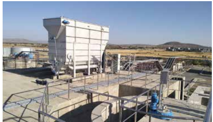
Bulbula IAIP WWTP 4000 CMD (2000 STP & 2000 ETP), Ethiopia
