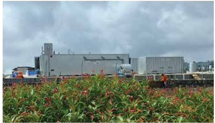
Selale University STP (2 MBR Packages) - Ethiopia Plant Capacity: 2000 m 3 /day
