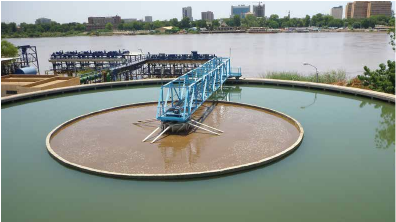
Pre-Treatment Plant for Dairy Effluent Emirates Dairy Farm 600 CMD, UAE
