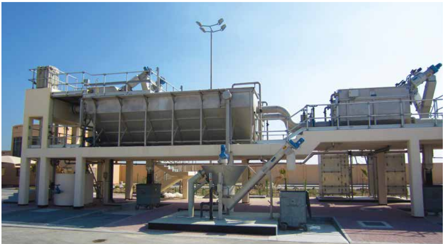
Ma'mir STP - Inlet Headworks with fine screen, grit & grease trap followed by membrane screen 2.215 m 3 /day, Bahrain
