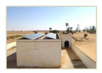
MENA-Water has now installed a photovoltaic solar pumping system whose 9.2 kW<sub>p</sub> power allows the operation of a DC borehole pump to provide an average of 72 m<sup>3</sup> of water per day. Next to supplying drinking water for habitants and travelers now as well it is possible to irrigate protective plants that provide food, shelter from storms and at the same time improve the local climate.
