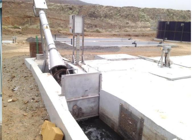
**Screening Channel for Tanker Discharge**
